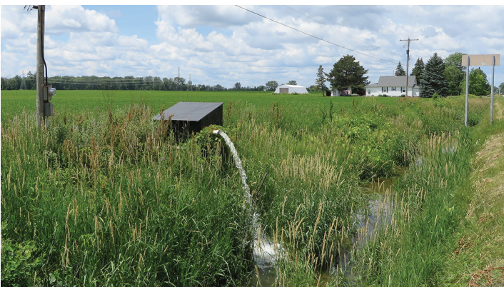
Figure 10- Top: Subsurface drainage outlet flowing into a drainage ditch that is at least 1 ft above the ditch bottom. Bottom: A relatively flat field with not enough grade to allow gravity flow of the drainage water into a drainage ditch, so the drainage discharge flows into a sump from which it is pumped out into the ditch.
